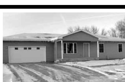
New Construction: 804 Jaxon $145,000
